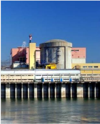
Refurbishment / Life Extension of Unit 1
