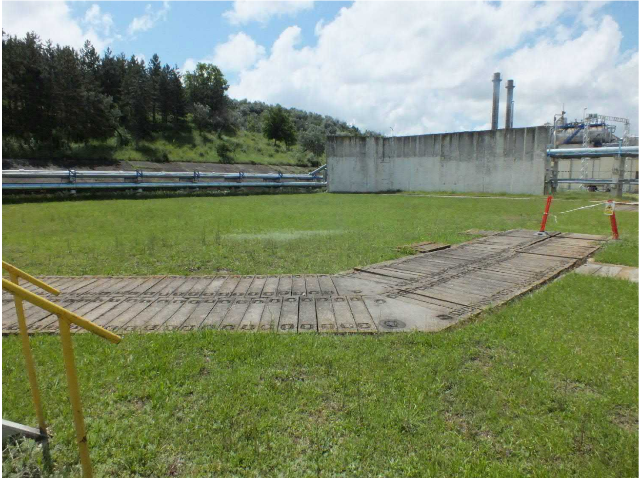
Figure 8-1: View of CTRF Project Site - Facing South
