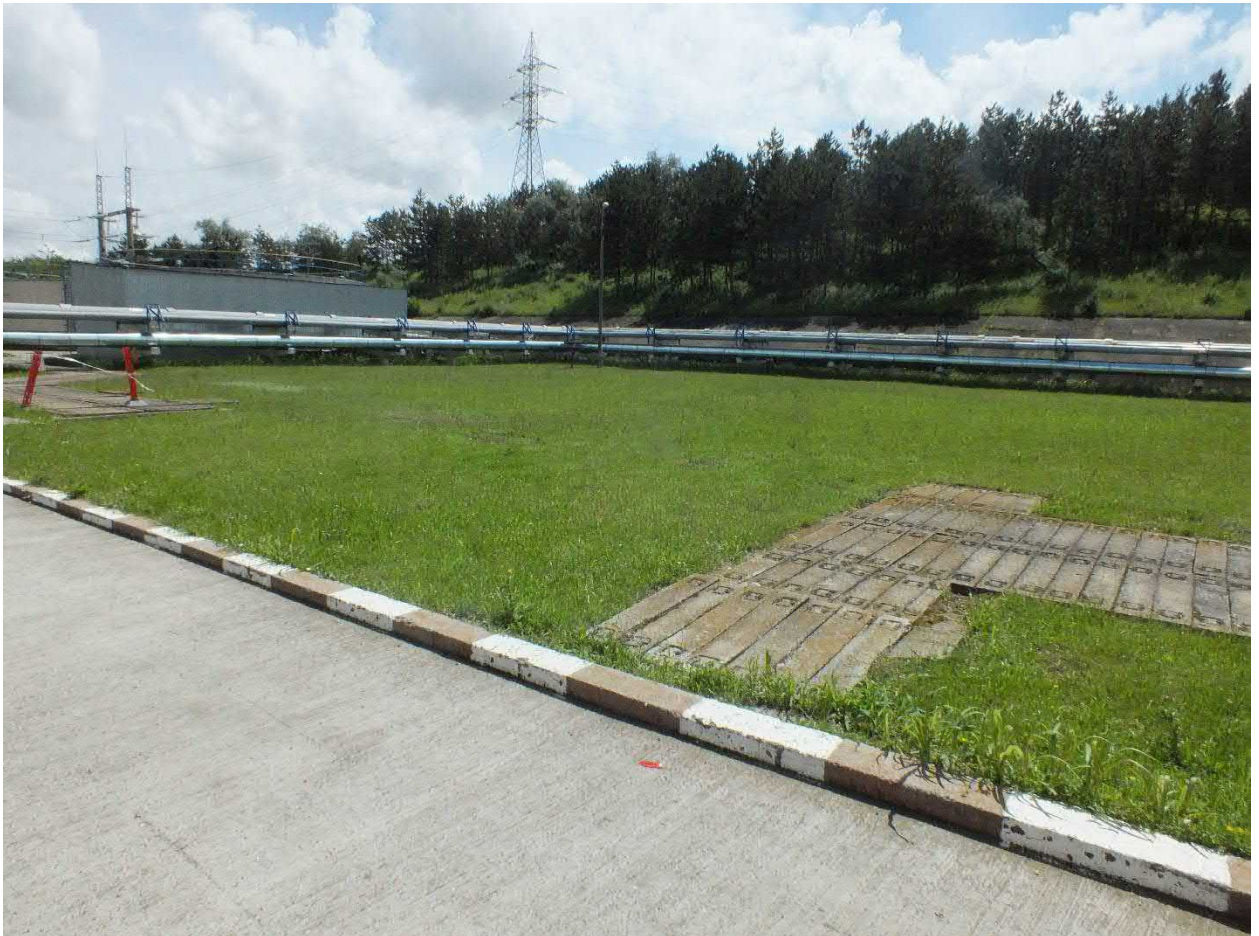
Figure 15-2: Photograph of the location of the planned CTRF, taken during site visit (17.06.2021)
